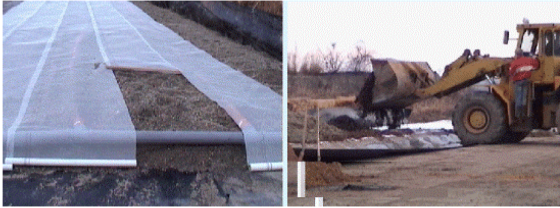
Fig. 1.21. Forming the pile with the drainage system
