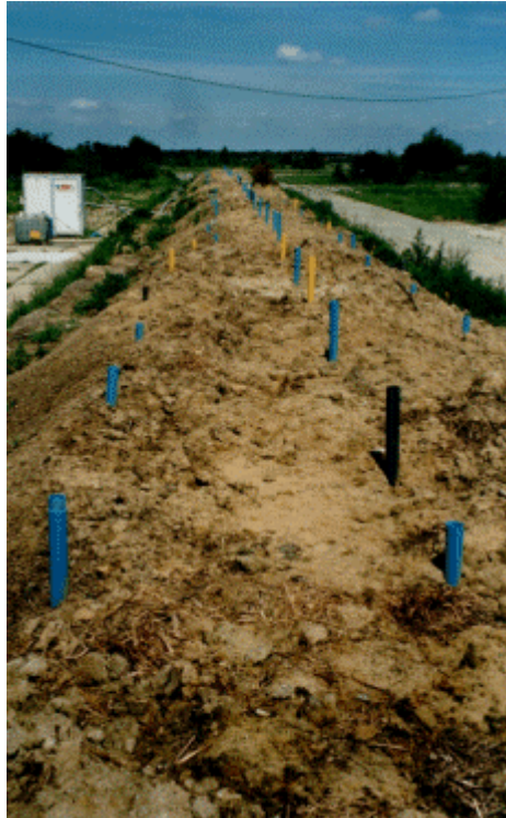
Fig. 1.15. Passive ventilation of the excavated ground using air lances
